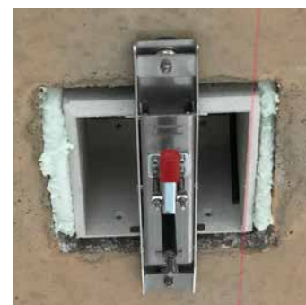
Airspot montage tool
